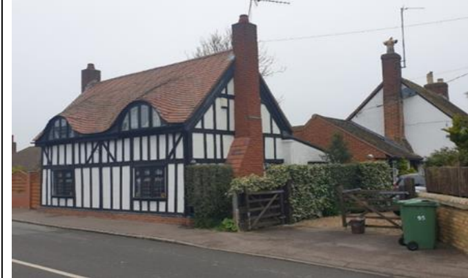
No 3 Mill Lane
