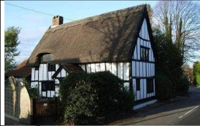
No. 154, Manor Road/Plumtree Cottage built 1609 with thatched roof and good example of eyebrow window.
