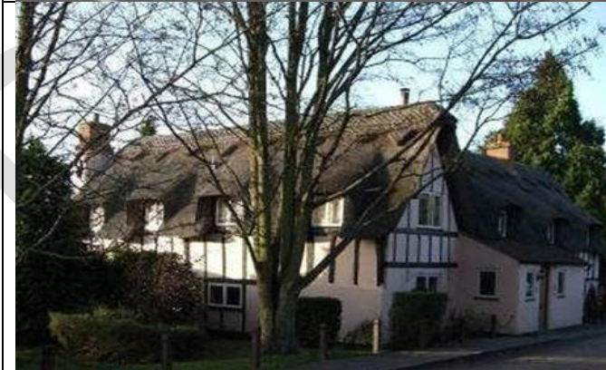
No. 8 Church Road. A good example of timber-framing with colour washed rough cast and thatched roof.
