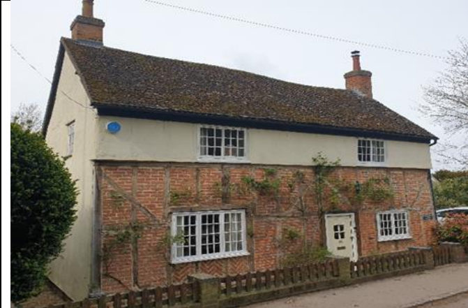
No 18 Church Road. A good example of timber-framing with brick inserts
