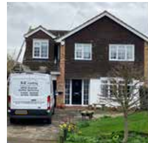
Mixed exterior finish including sand brick, render and brown tiles. Also features intersecting gable roof and gable dormer.
