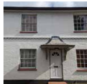
Painted Flemish bond brick work with decorative course. Gridded sash windows and deco porch.
