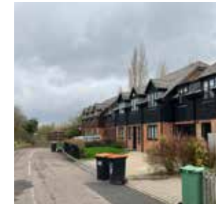
Rare mix of red brick and black weatherboard. Ample setbacks for driveways and lawns. Features slate tile roof with gable dormers.
