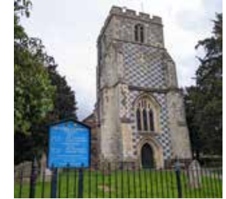
St Nicholas Church with a distinct battlement roof and flint and limestone chequerwork.
