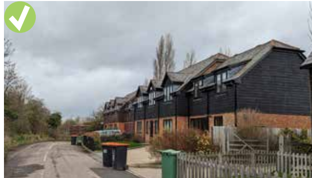
Figure 51: Local example of a south facing property (approx. 30 degrees) that maximises the solar gain, while plantation to the north offers protection from cold northerly winds.
