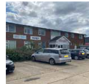
Gable porch with uPVC windows. Main building featuring a flat roof.
