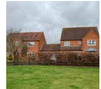
Picket fence, hedgerows and trees used as boundary treatments while allowing for transparency of use.
