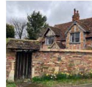
Red brick garden wall with lychgate. Facade with mix of Flemish and stretcher bond brick work. Gable fronts with timber frames.
