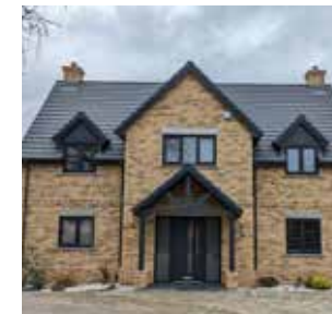
Contemporary detached house with slate tile roofs, weatherboarding finish on gable dormers and a dormer porch. Sand brick is used with brick course detailing.
