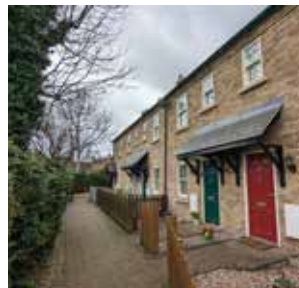
Contemporary mews with sensitive exterior finishes such as brick stretcher-bond and wooden sash windows.
