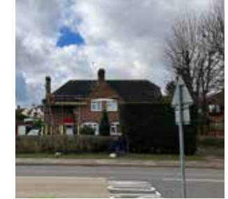
Semi-detached house with a shared gable front and a mix of hipped and jerkinhead roofs.
