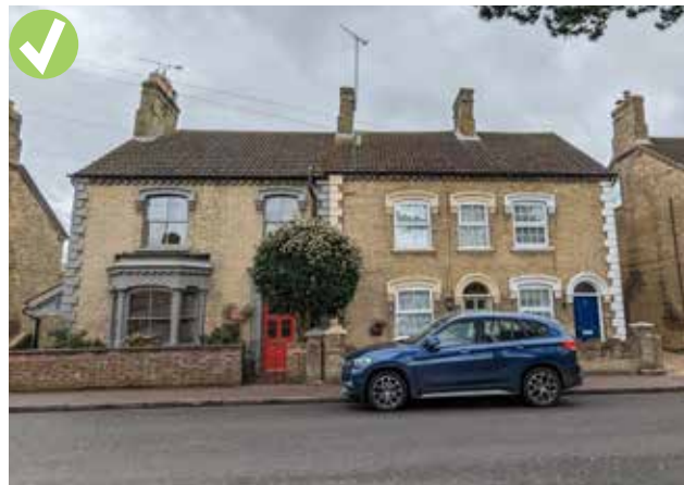
Figure 52: Local example of terraced housing. This typology provides more efficient envelopes compared to semi-detached or detached houses.
