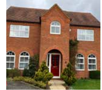
Red brick detached house with corbel detailing, wide rounded lintels and a prominent porch.
