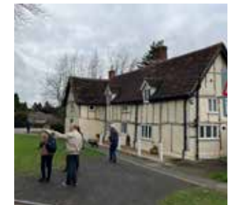
Elm Tree Cottage with T-plan, clay tile roof, off cast render and timber frame. Small gable dormers feature wooden casement windows.
