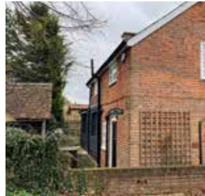
Flemish bond red brick, with black weatherboard extension. Wooden casement windows.
