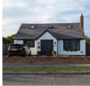
Renovations add to the local vernacular, providing a more contemporary feel.
