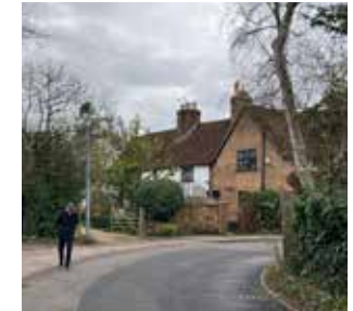
Barton Manor with mixed red brick, clay roof tiles and white render exterior finishes.
