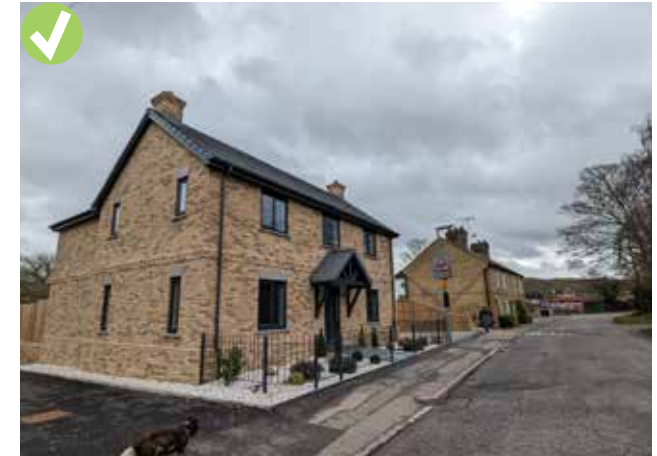
Figure 22: Local example of a positive infill development which matches the surrounding context in the figure 23 below.
