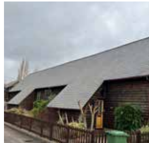
Distinct row of terraced houses with wide front facing porch set within a slate tile catslide roof. Rare use of weatherboarding.
