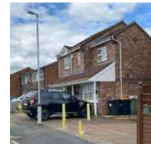
More contemporary architectural styles stand out among later 20th Century properties. Primary use of brick and clay roof tiles provide the distinction.
