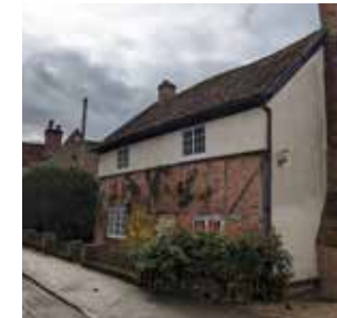
17th Century cottage with timber frame and colourwashed brick nogging.
