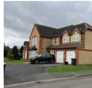
Large detached house with hipped roof and intersecting gable. Also features internal garage and bay windows.
