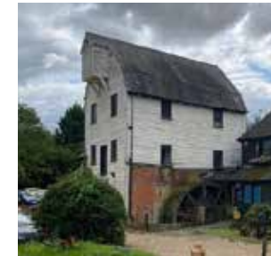
White weatherboarding with gridded black windows. Projecting hoist previously used for industrial purposes.
