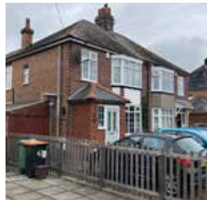
Early post-war semi-detached house with hipped tiled roof and bay windows. Additional Hipped porch extension.
