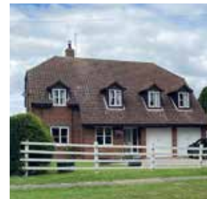
Use of black weatherboard for small pitched dormers and the rare use of a catslide jerkinhead roof.
