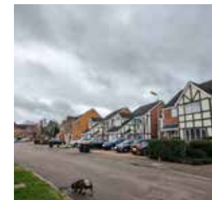
Infrequent clusters of mock Tudor style with timber framing and render mixed with redbrick. A further example of slate tile catslide roof.
