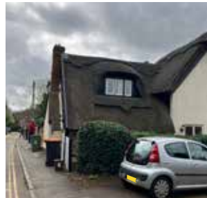
Example of thatched roof with decorative ridges and eyebrow dormer.
