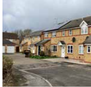
Semi-detached houses arranged at the end of a cul-de-sac. Light brick with red brick course and quoin detailing.
