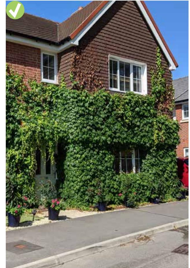
Figure 53: Example of a property with vegetation of the facade, elsewhere in UK.
