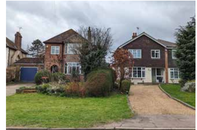
Figure 08: Local example of detached houses.
