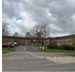
Higher density housing, including maisonettes and terraces, in a typical post-war style.
