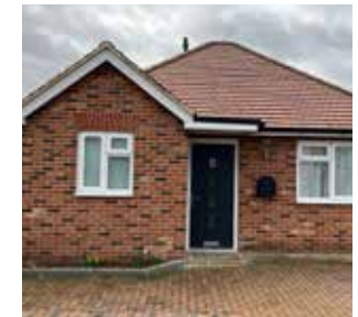
Contemporary bungalow with hipped, red clay tile roof and protruding gable front.
