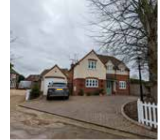
Contemporary house that contrasts with the area's primary typology. Features gable dormers, jerkinhead roof and curved lintels.
