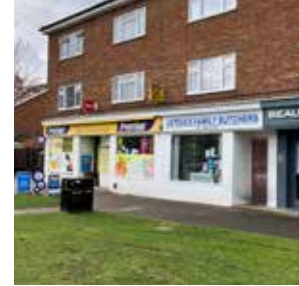
Ground floor shopfronts of differing styles along the shopping parade. Above floors with brown brick and uPVC casement windows.
