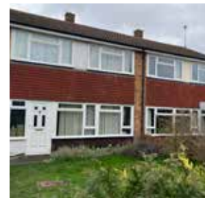
Varied facade treatments including red tiles, brick, weatherboarding and render.
