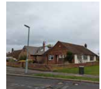
Bungalow with intersecting pitched roof and low brick wall boundary treatments. Additionally features clay tile roof and red brick exterior finish.
