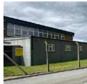
Corrugated steel facade treatments on extension to a more prominent office building.
