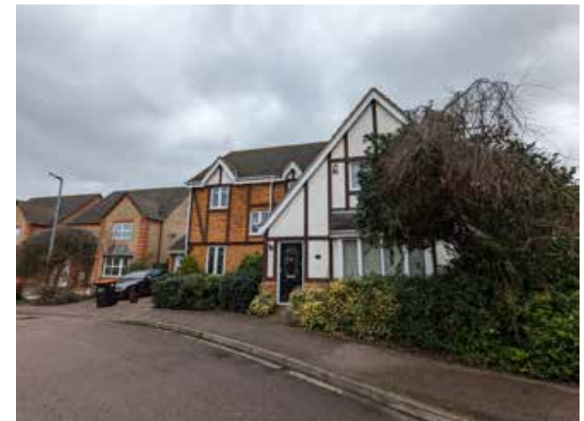
Figure 05: Positive example of development that enhances the local vernacular of the area: timber frame with render and brick infills.
