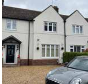
Semi-detached houses with render and red brick plinth base. Also features pitched roof with adjoining intersecting gable.
