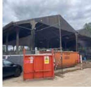
Exposed warehouse with corrugated steel pitched roof.
