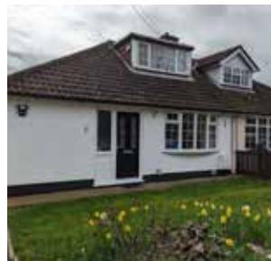
Hipped, clay pantiled roof with dormer and gable dormer windows. Render finish with weatherboarding and casement windows.
