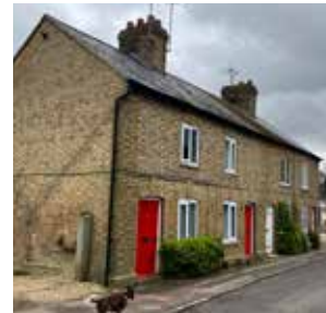
Brick terrace houses with pitched slate roof and curved lintels above front doors and ground floor windows.
