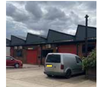
Sawtooth roof style with gridded casement windows. A light industrial building featuring more architectural interest.
