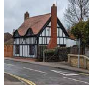
Cottage with white render and Tudoresque black timber framing. Features a pitched roof with eyelid dormers and clay tiles.
