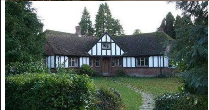
No. 52, Hexton Road. A good example of a Victorian Butterfly Plan style property.
